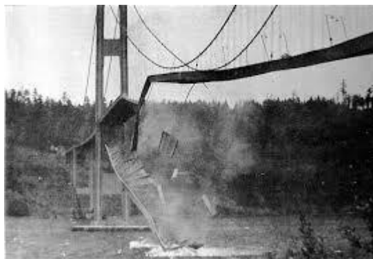
Figure 3: Crash of the bridge due to wind-induced vibrations.
